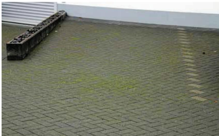
**Fig. 13b:** ... owing to insufficient cleaning of the joints between concrete pavers
