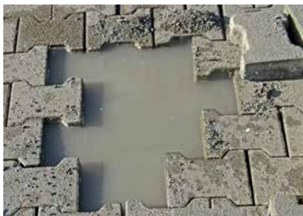
**Fig. 9: Insufficient water permeability of the base course or subgrade**
