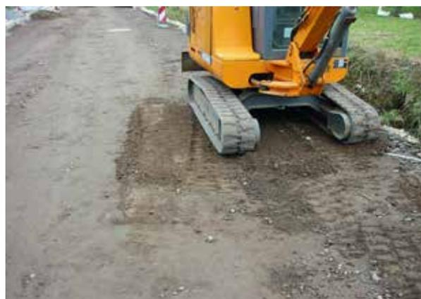
**Fig. 10: Soiling and/or consolidation of the base course**
